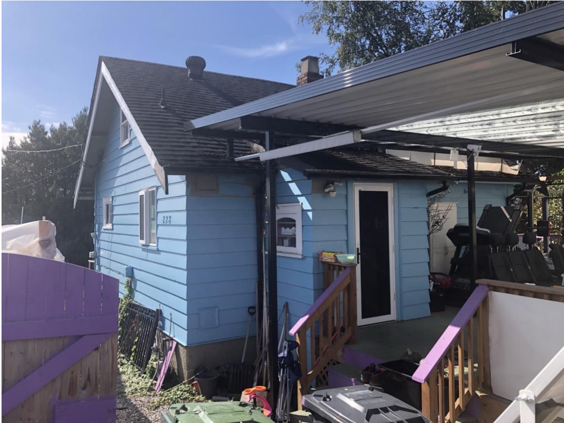
Figure 8: Rear of 228 Thrift Street: note that the main floor is nearly at ground level here due to the slope of the property.
