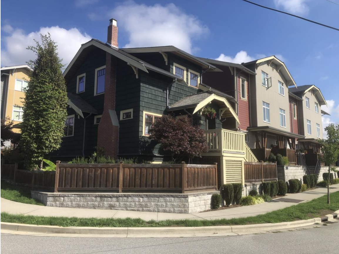
Figure 13: 801 Roderick Avenue – Rocheleau Cottage (1929) integrated with townhouses (2015)
