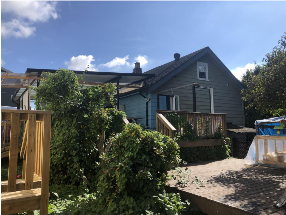
Figure 9: West side of 228 Thrift Street.
