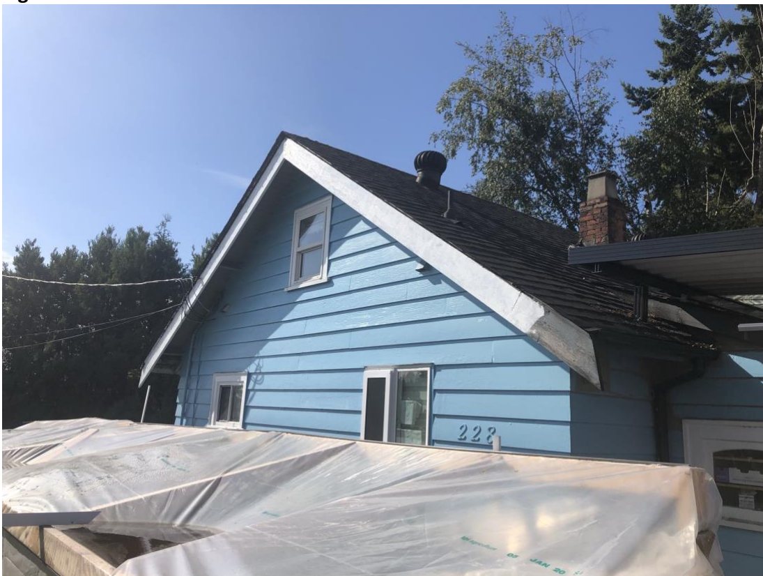
Figure 7: East side (upper portion) of 228 Thrift Street
