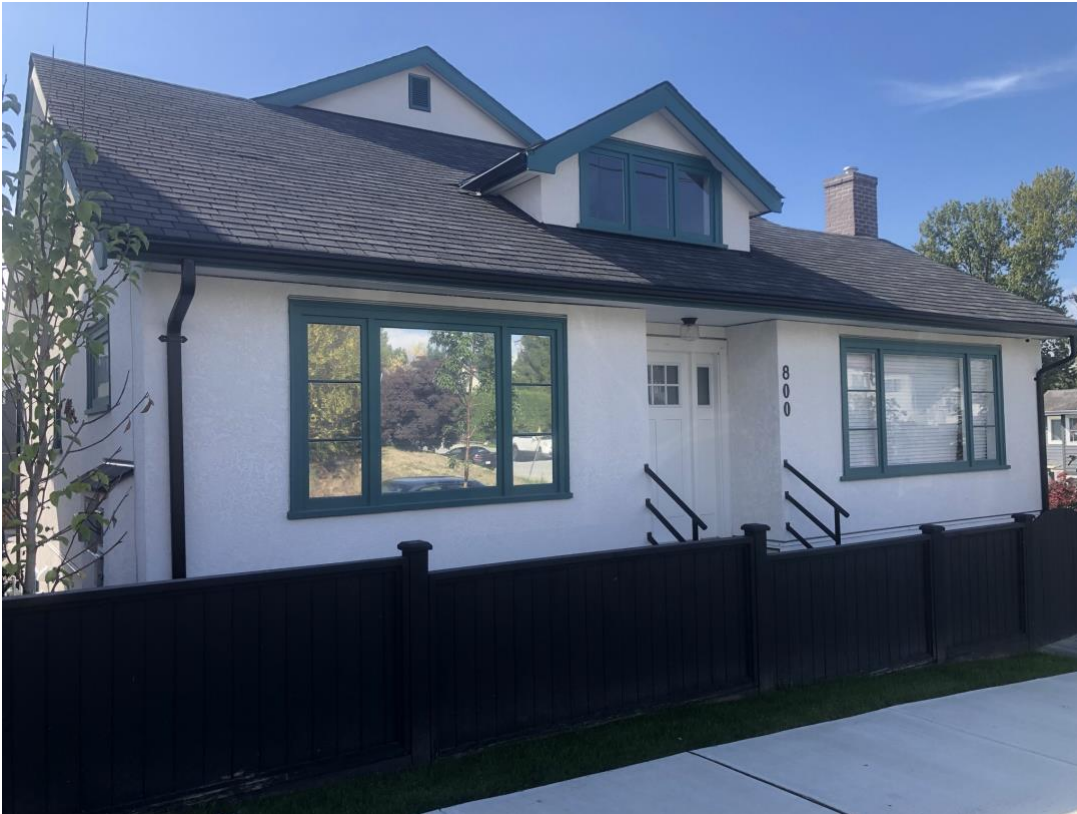
Figure 14: 800 Gauthier Avenue, Prost House (1944)
