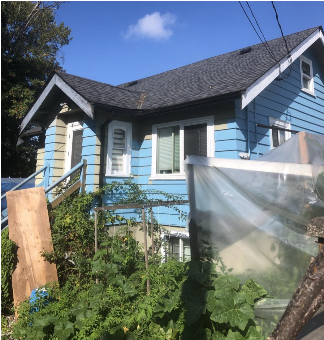
Figure 5: Front of 228 Thrift Street, with the front porch facing Lougheed Highway and significant hedge providing a buffer to the busy thoroughfare.
