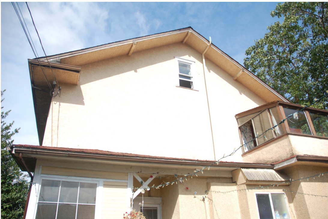
Rear with enclosed lower porch and enclosed second floor porch
