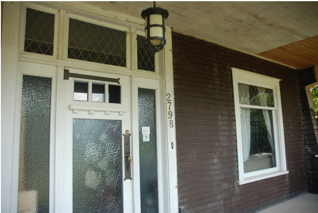
Main entry with transom and sidelights; rear door to upper porch with inset leaded glass transom
