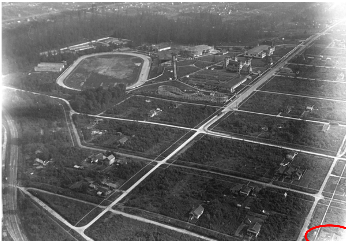
Aerial View of Hastings Park and Racetrack, Streetcar Line and Nearby Houses. CVA 1123-1 Race Track - [Hastings] Park, 1919. 2798 Yale Street at bottom right corner.
