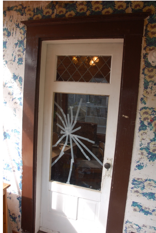
Rear door to enclosed porch
