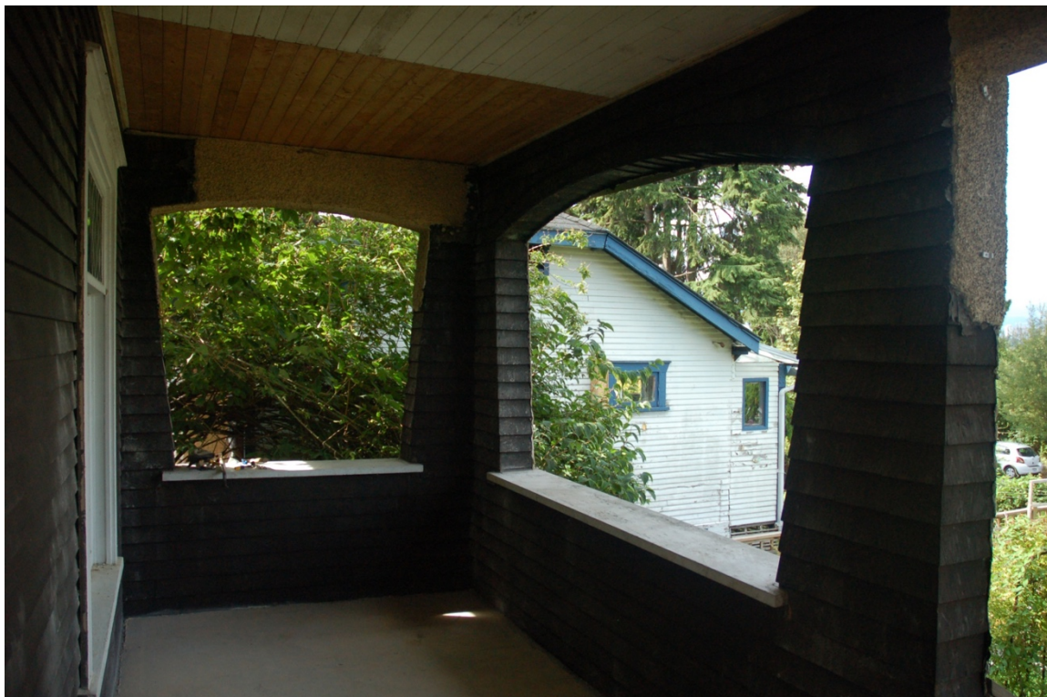
Front porch interior detail (original shingles)
