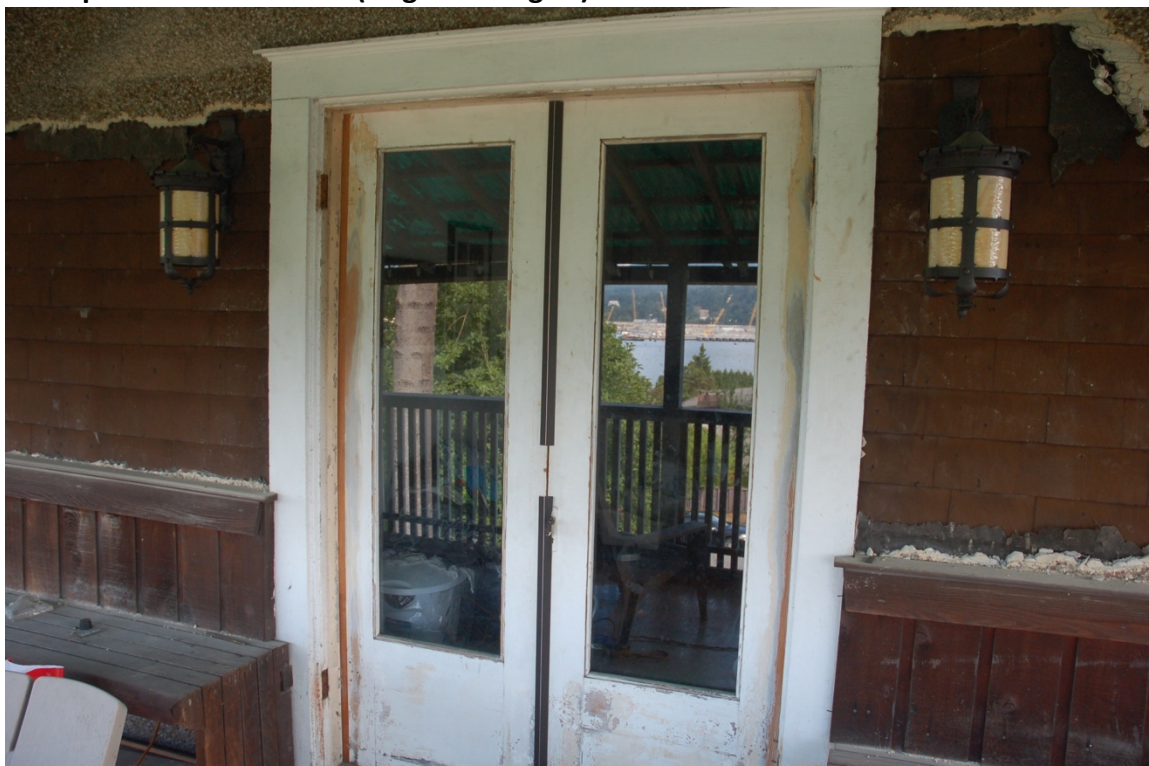
Paired doors to upper porch with exposed original shingle cladding
