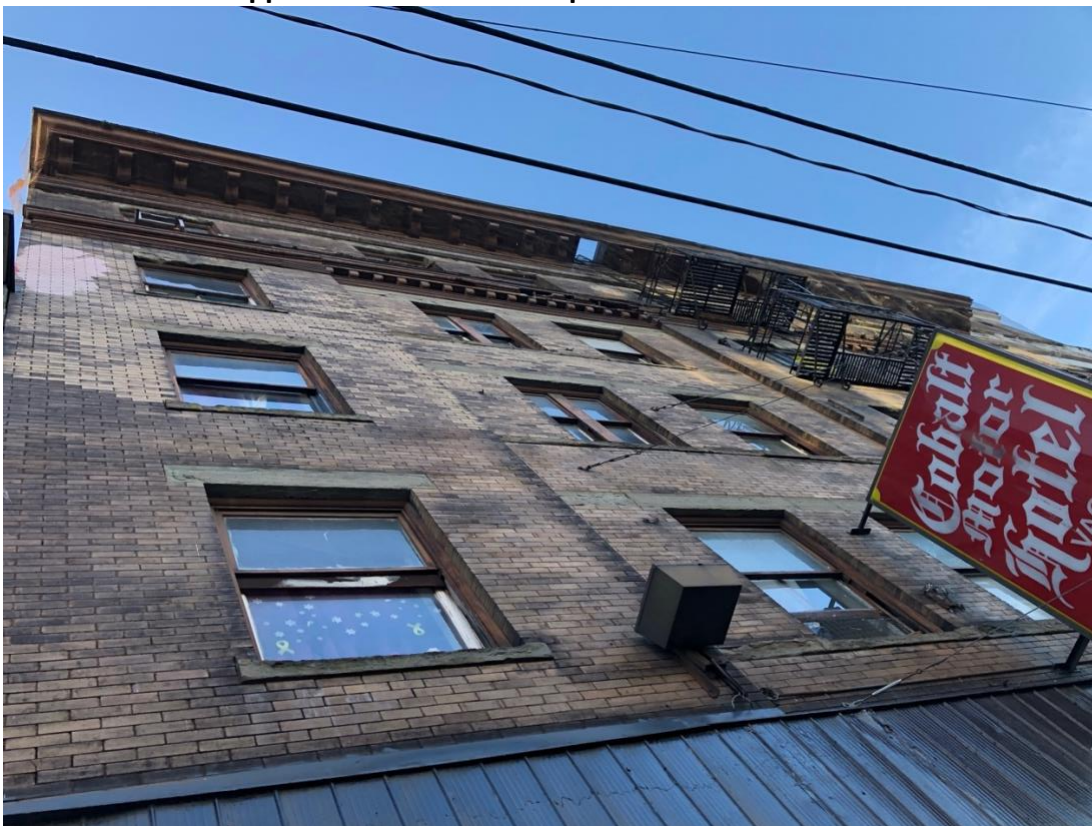
Front elevation - upper floors and signage.
