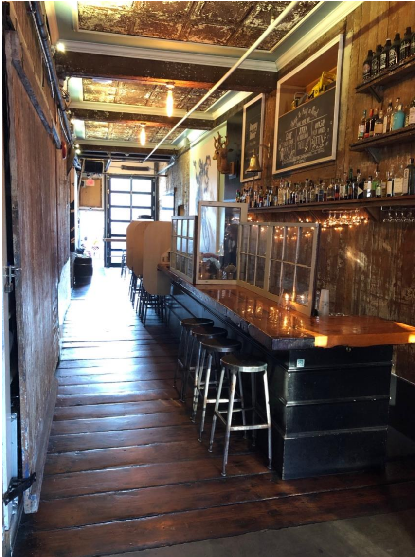
Original pass-through from street to rear of site, featuring a number of original, early or historically compatible components including pressed tin ceiling, timber cross-connections, rough wood walls and heavy timber flooring.
