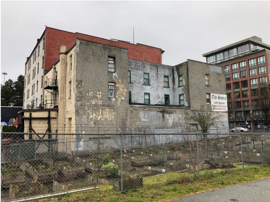
South Elevation – Cobalt Hotel displaying painted red wall.
