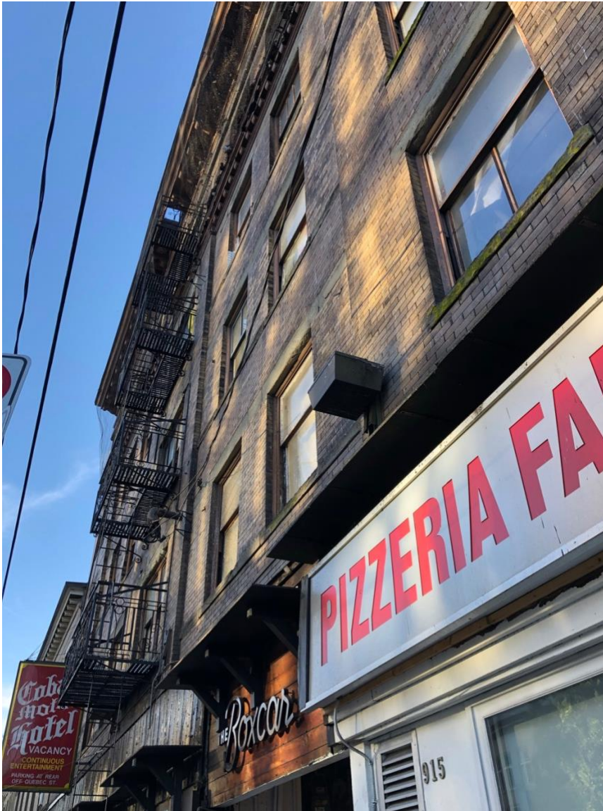
Partial view of storefronts and upper floors.
