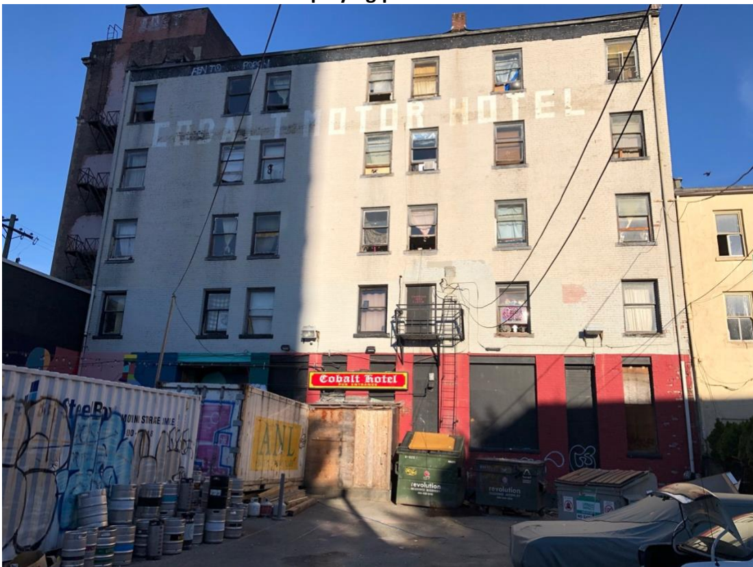
Rear Elevation (west side).
