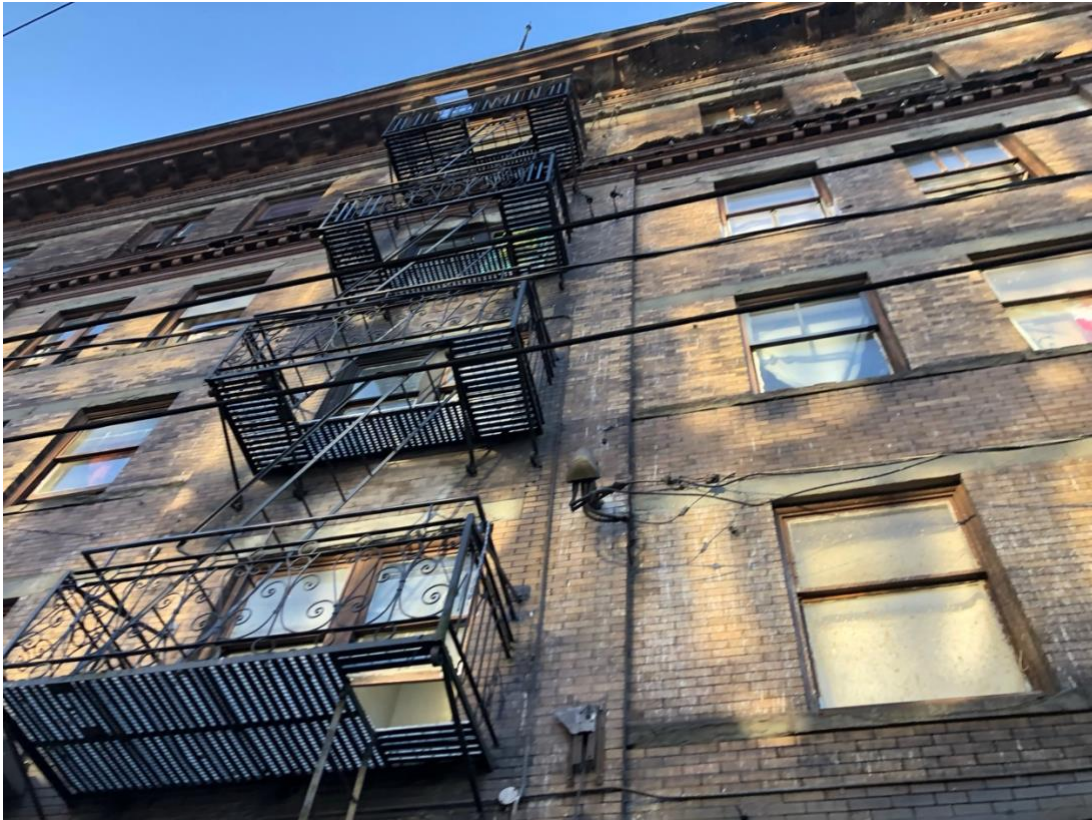
Front elevation - upper floors and fire escape.
