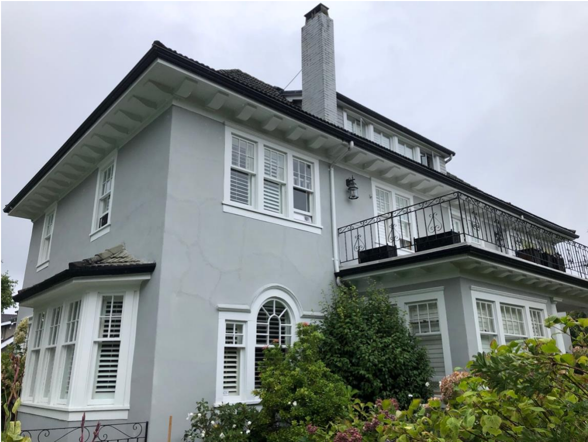
Figure 10a: East side – Front entry not visible, see photo below
