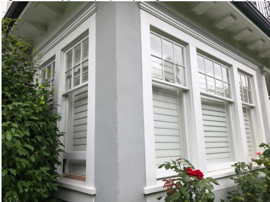
Figure 23: Front room adjacent entry porch
