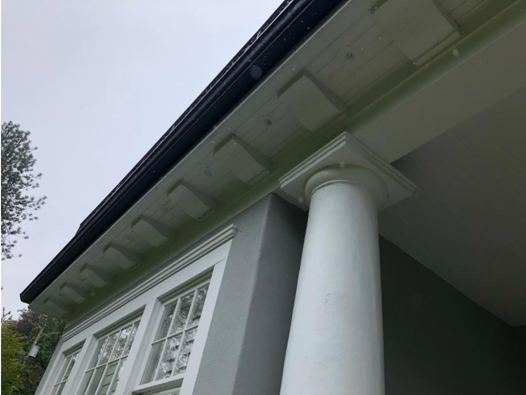
Figure 25: Detail of curved brackets in soffit
